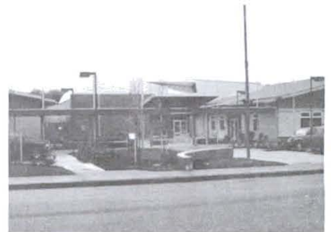
The entrance to the City Services Center, at 21630 11th Ave. S. has been reconstructed.
